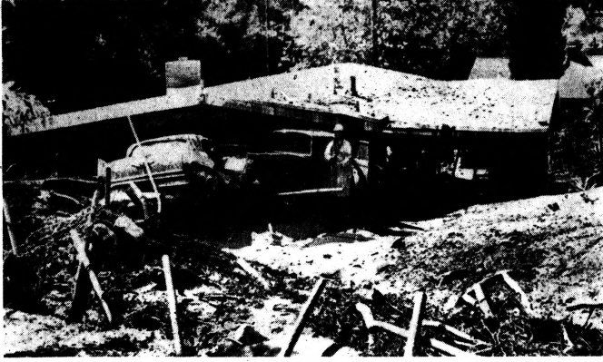
SMASHED BY MUD — A sliding wall of earth and water washed through this canyon above Burbank, Calif., yesterday, leaving a path of destruction behind and one person missing.
