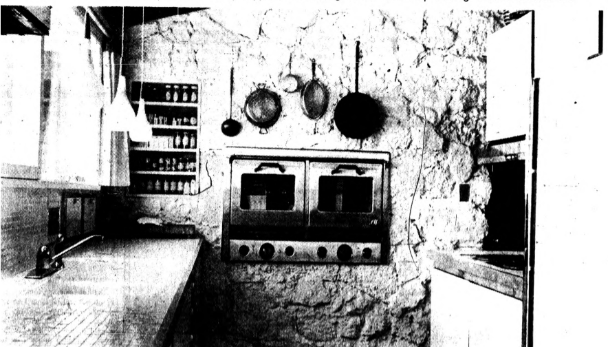
Broken Sidewalk Concrete, Rough Side Out, Is Mounted On Sidewall Of Country-Modern Kitchen
