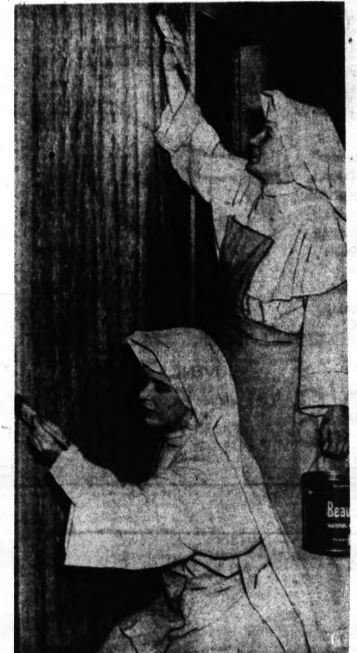
PUTTING FINISHES — Putting final touches of wood finish on the dining room walls in the Dominican Sisters' new retreat house in Oxford Township are, from left, Sister William Marie and Sister John Marie. The nuns and novices did all the sanding, painting, decorating and even the tiling of floors.
