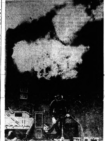
WALL CAME TUMBLING DOWN—Seconds after Indianapolis Star photographer Bob Daugherty took this picture, the east wall of the Lindeman Wood Finish Co. collapsed. The Sunday afternoon blaze destroyed the three-story brick building, causing damage estimated in excess of $150,000. Firemen in foreground prepared to leap to safety when exploding paint and lacquer drums caused the ball of fire which broke through the wall. No one was injured.
