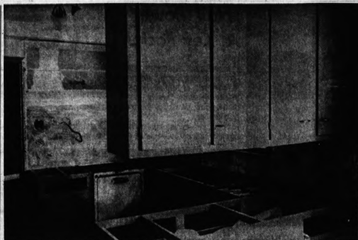
FROM CHAOS—In the stage of remodeling, the kitchen of the John Greenleys, 2803 Mackintosh, Bloomfield Township, was hardly an ideal work center. But Bloomfield Custom Kitchens of 4068 W. Maple, Bloomfield Township, would soon wave the wand of work and create an answer to a homemaker's dream.
