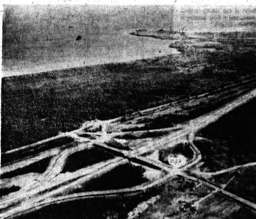
NEW INTERCHANGE —Morsehoe Bay, at top of Lake Huron, and lush Upper Peninsula forests surround this new Interstate 75 interchange at M123 north of St. Ignace. Comple-
