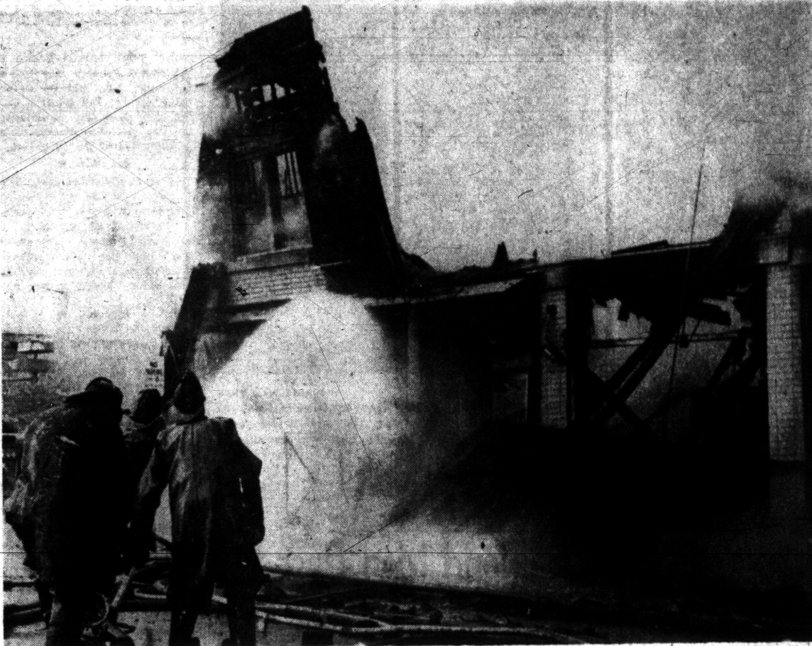
BUSINESS CORNER HIT — All that remains of the second-story apartment in which a 70-year-old Royal Oak man suffocated this morning is a jagged piece of wall. The upstairs portion of the building collapsed at the height of the blaze and the body of Patrick Seward was found two hours later in the ruins downstairs.
