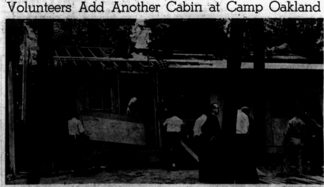
BUILDING BEE — Part of the 80 DeVlieg Machine Co. employees who joined in a building bee Saturday at Camp Oakland are shown as they rush construction of a 38 x 18-foot cabin which will house groups of children for two week summer vacations. Employees of the Ferndale company started work at 5 a. m. and hoped to finish by dark but rain delayed completion of the project. The volunteer workers, who supplied all their own construction materials, said they would finish the job next Saturday. Camp Oakland on E. Drahter road about one mile south of Oxford is under the jurisdiction of Oakland County Juvenile Court.
