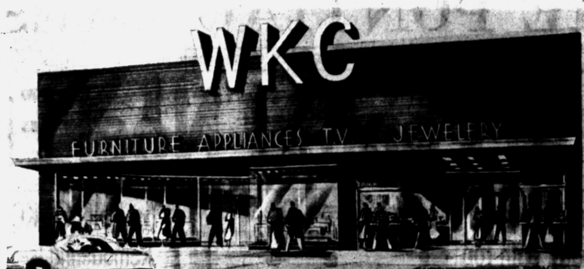
NEW FACE—Sporting a brand-new look is the WK&C store at 108 N. Saginaw St., which has just had its "face" lifted. Used in the construction of the 72-foot-wide front were Italian marble, extruded aluminum and a special Virginia brick, according to J. J. Walinger, store president. The second phase of the store's remodeling program is slated to get under way in January and will feature changes to the store interior.
