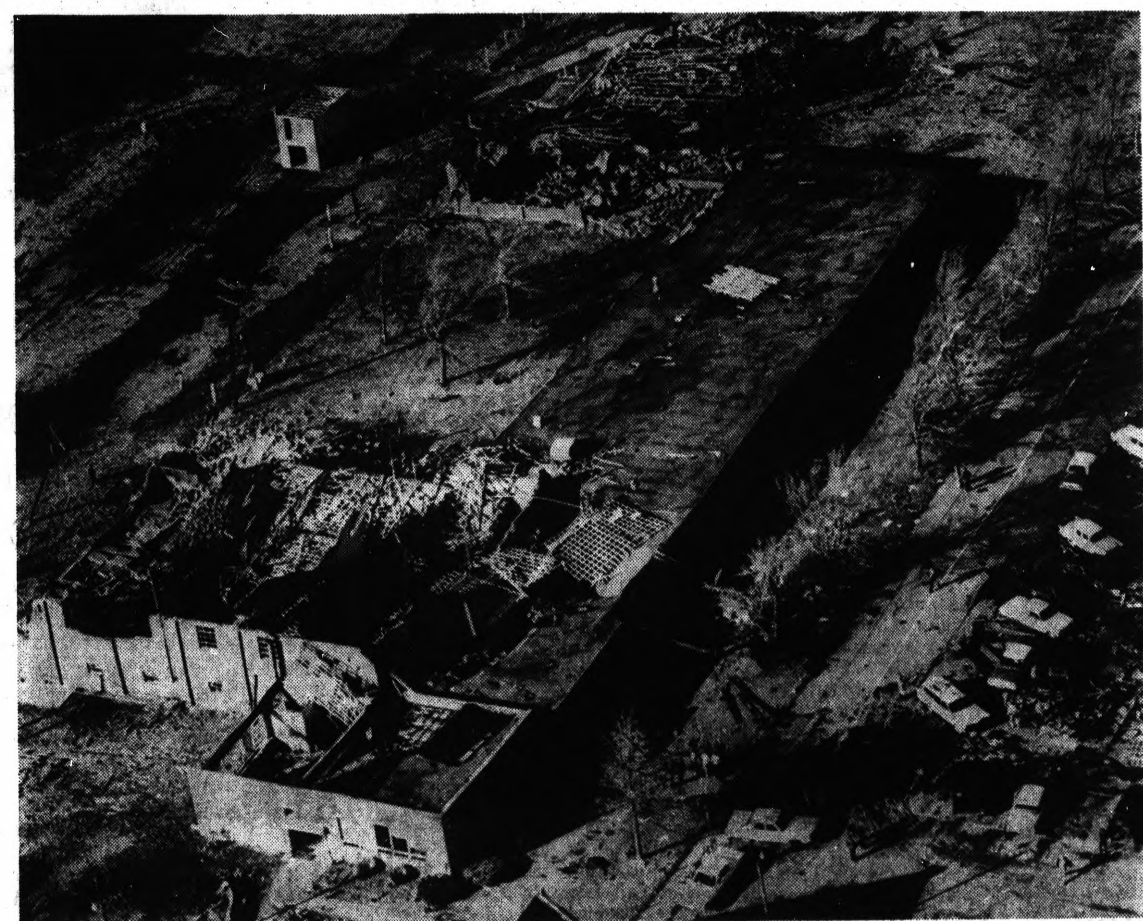
Wrecked Shell Remains After Tornado Hit Orrick, Mo., High School
