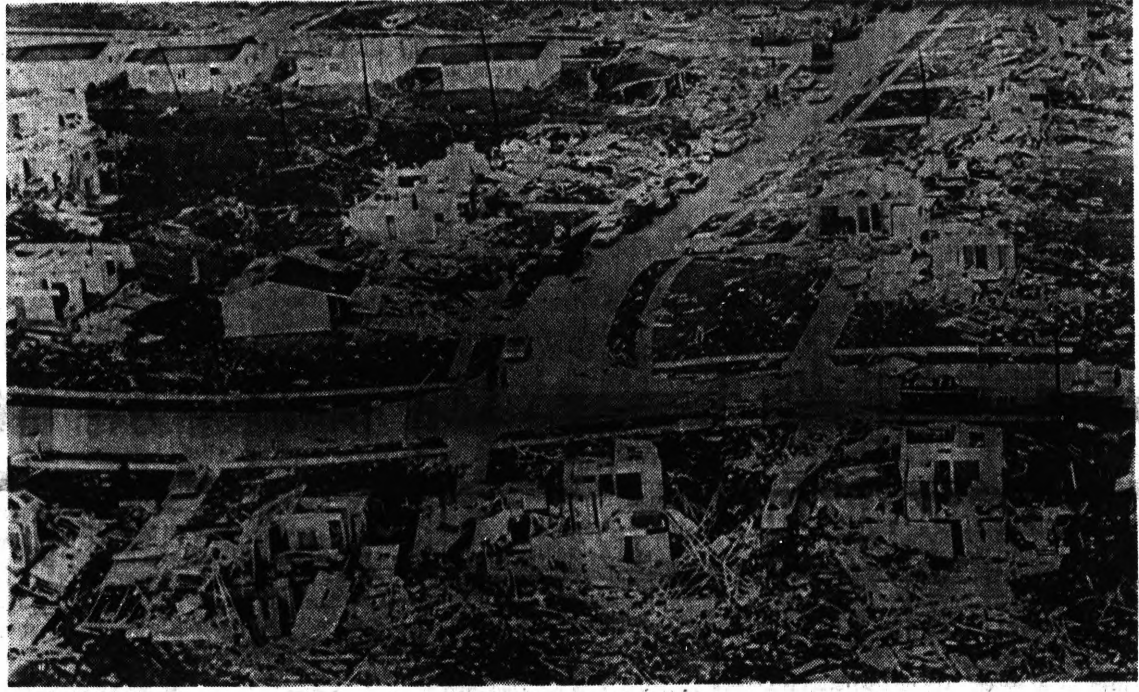
Debris Literally Blankets The Ground In Maryland Heights, Mo.
