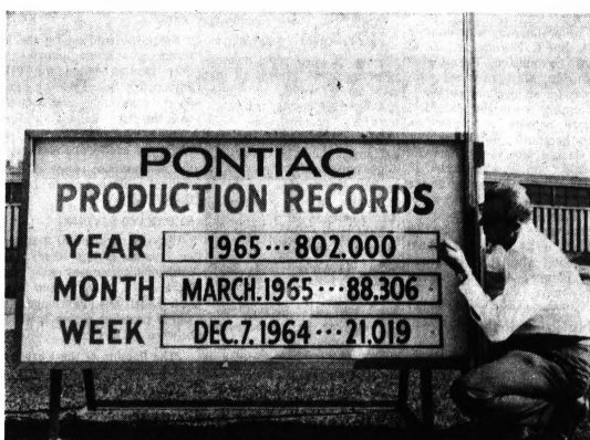
ANOTHER RECORD —Pontiac Motor Division early this morning closed out its 1965 model run with an all-time record of 802,000 cars. Substituting the new figure in a sign atop the plant protection booth at the main
