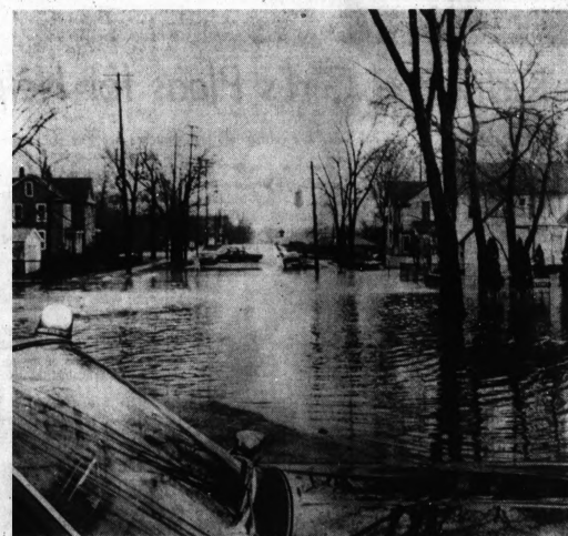
FLOODED STREETS — This morning scene at Sanderson and Augusta was repeated in many areas in Pontiac today. A great number of home owners found today that their basements had a similar look.
