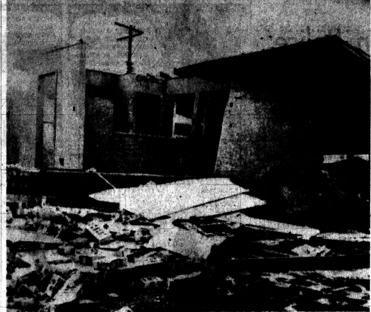
WREAK HAVOC — Roaring winds dismantled several homes like this one in the Ogden, Utah, area early yesterday. The 80 mile-an-hour winds collapsed a wall of a Baptist Church, uprooted trees and felled power lines throughout the second largest city in Utah.
