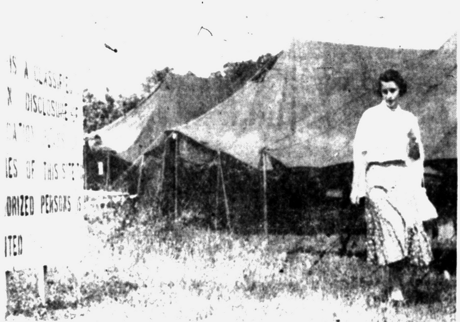
SECRET SITE — An unidentified government worker stands post the tents at the secret center today in the simulated atomic attack on the Capitol near a sign which denotes the area as "classified." President Eisenhower and his key aides were following relocation of government operations yesterday in similar tents at the site.
