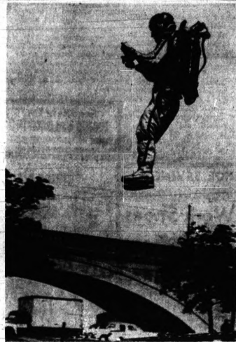
NO TRAFFIC — Harold Graham floats through the air to demonstrate one way for pedestrians to fight back on busy streets. The rocket belt, developed for the Army, was shown in Boston. Graham traveled 120 feet in 15 seconds at a maximum height of 20 feet.
