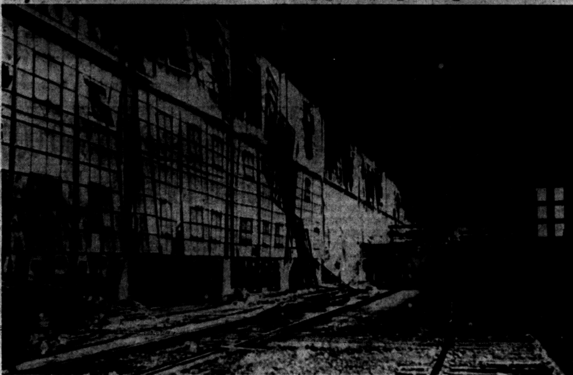
BLAST DAMAGE — A 500-foot section of Dearborn's giant Rouge plant of the Ford Motor Co. stands twisted and torn following an explosion in the paint spray section which injured 22 workers last night. Although the cause of the blast was not immediately known, it was believed to have originated in a huge paint-drying oven.
