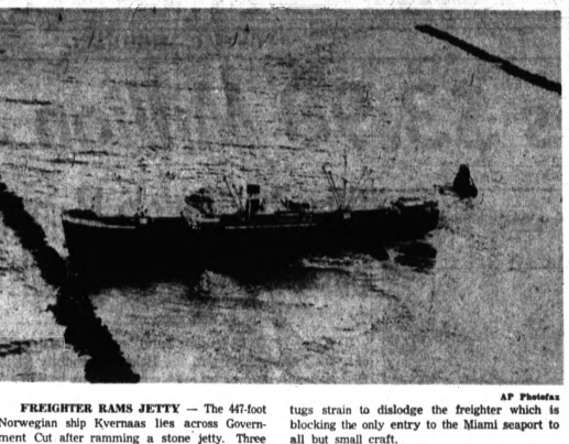
FREIGHTER RAMS JETTY —The 447-foot Norwegian ship Kvernnaas lies across Government Cut after ramming a stone jetty. Three tugs strain to dislodge the freighter which is blocking the only entry to the Miami seaport to all but small craft.
