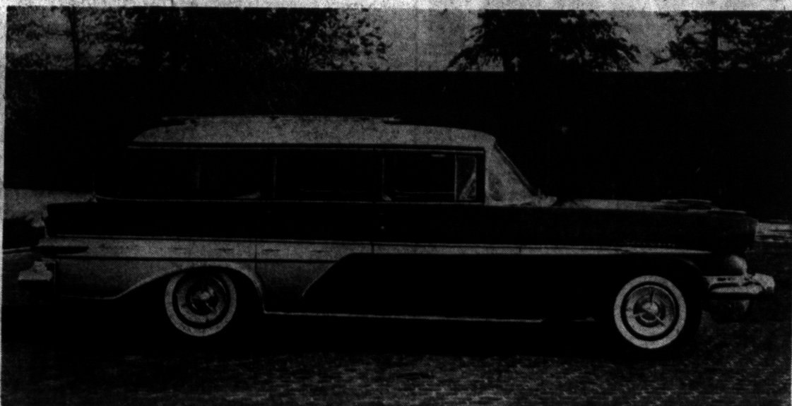
THE CUSTOM SAFARI — A reclining right front seat is one of the features of the Pontiac Star Chief transcontinental Safari, scheduled to make its debut in New York this week. Powered by Pontiac's new V8 engine with triple two-barrel carburetors, the station wagon is a production model which will go on sale at Pontiac dealerships early in 1957.
