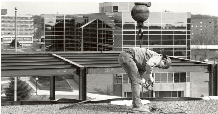
Kresge Library Renovation, 1966
