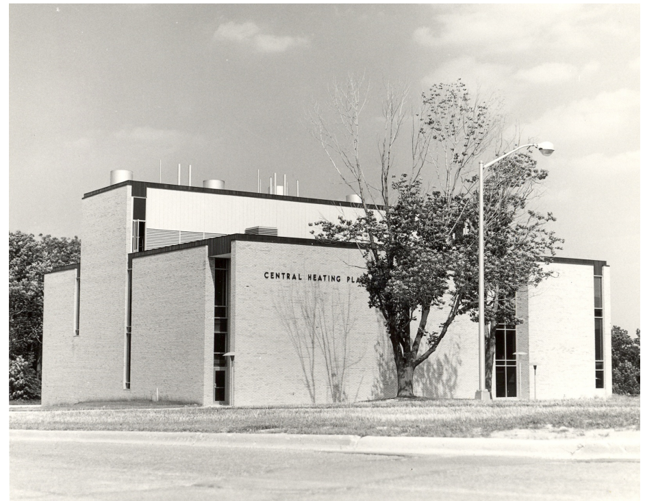
Central Heating Plant, 1966
