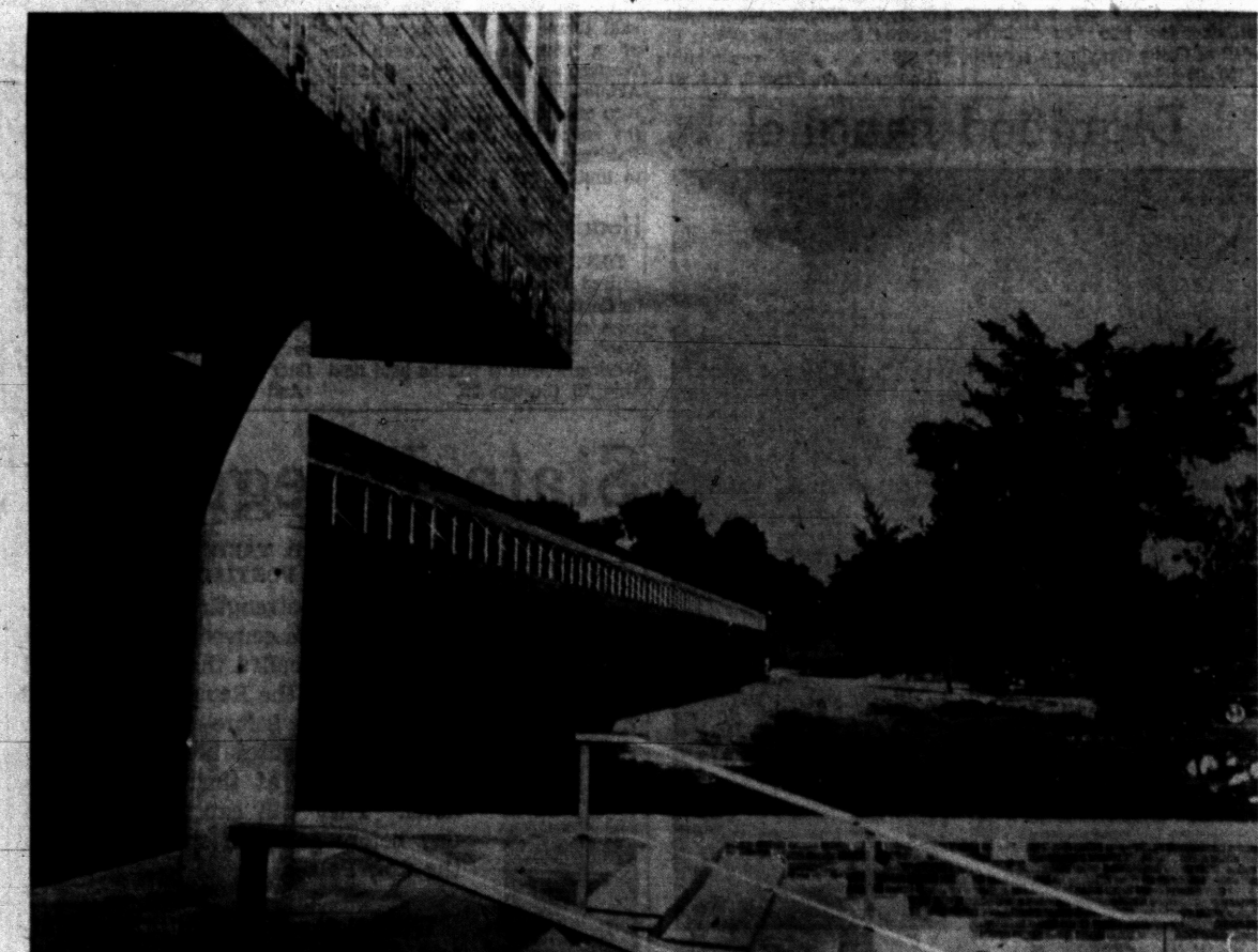
STRETCH OF CLASSROOMS—New addition at Birmingham High School, seen from the main steps, will be open when students report for classes on Sept. 6. Housing 11 classrooms, it features
