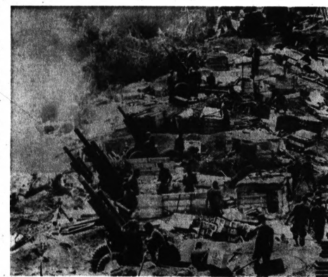
MUSCLE FOR MARINES — A Marine artillery unit digs in its 160mm howitzers west of Hue as a fire support base for troops sweeping the area. Troops carved and blasted away the jungle all day to prepare the gun pits and bunkers.
