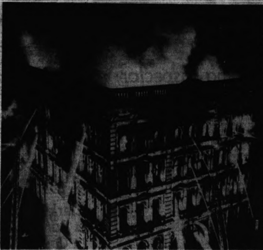
IN DOWNTOWN NEW YORK — Flames raged through this five-story loft building in downtown New York Friday night. Three firemen died, trapped in the basement by flames that cut off their escape route. The belching black smoke could be seen for miles. The 100-year-old brick building housed textiles. Some 350 firemen were on the job before the blaze was finally brought under control.
