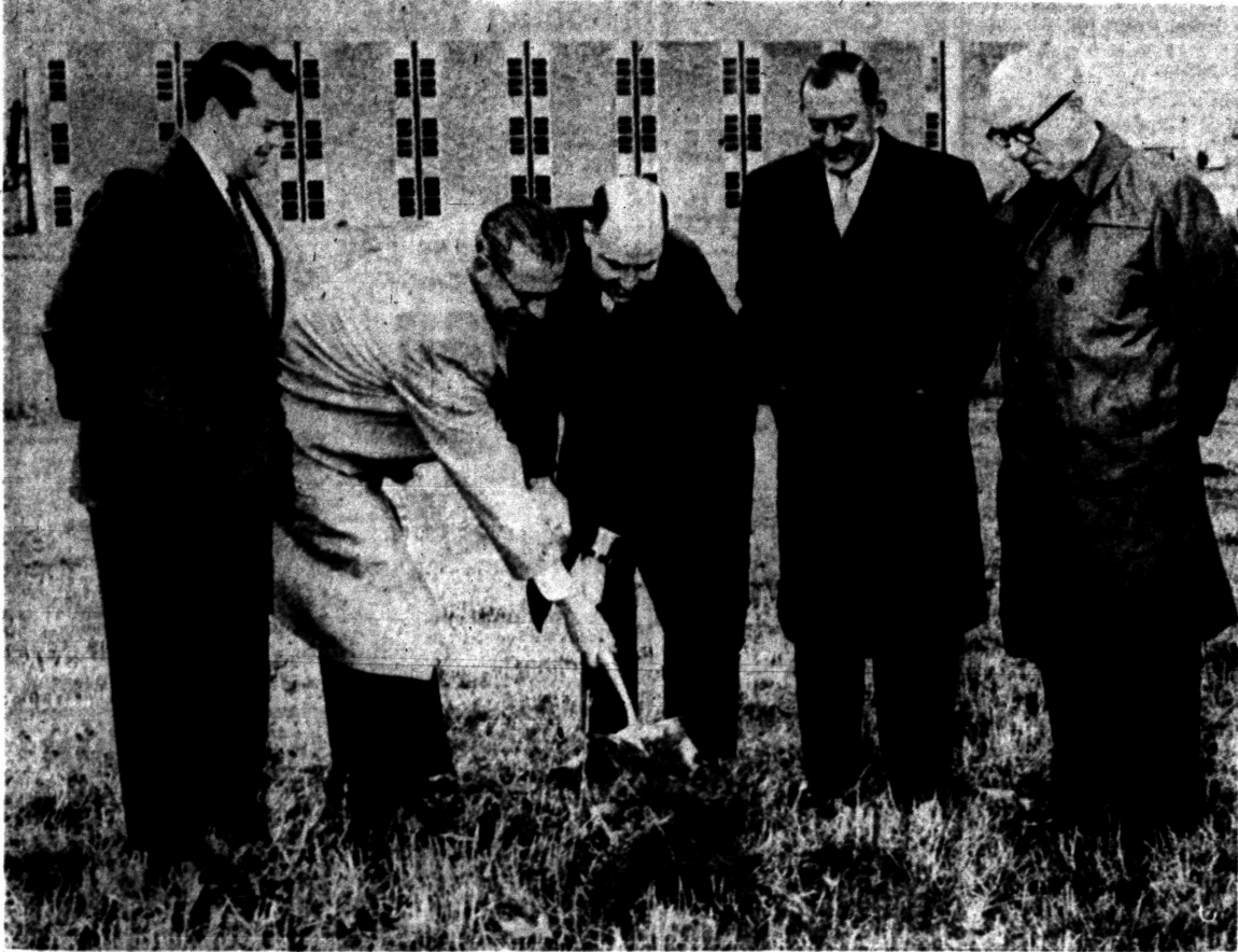
STUDENT CENTER GOING UP —Ground-breaking ceremonies for Michigan State University Oakland's Student Center were held this morning. Digging the first earth aside are Delos Hamlin (left), chairman of the Oakland County Board of Supervisors, and MSUO Chancellor D. B. Varner. On the left of the shovelers is Roy Alexander, director of student services. Also watching are Harold A. Fitzgerald, Pontiac Press publisher, and Alfred C. Girard (far right), president of the Community National Bank. In the background is MSUO's first academic building.
