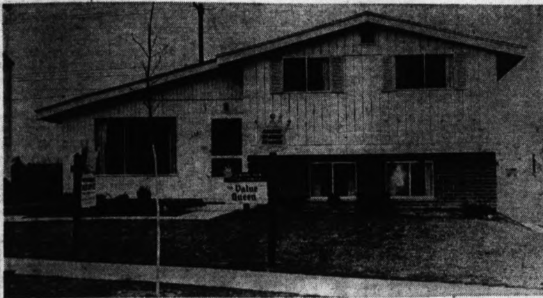
PONTIAC KNOLLS — Four bedrooms and a compartmented tile bath are a feature in this tri-level house, the Value Queen, located at 114 Victory Drive, in Pontiac Knolls. There is a finished activities room and a half bath on the lower level. A large living room and kitchen
