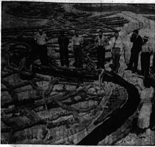
DOWN THE MISSISSIPPI —These folks are standing near Angola, La. Rather, they are standing where it is represented on this miniature scale model of the Mississippi River. The layout was made by the U.S. Army Corps of Engineers at their Waterways Experiment
