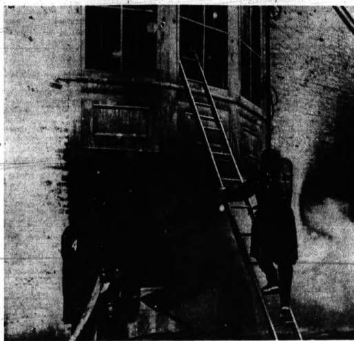
FIGHTING BLAZE—Firemen are shown entering the Orchard Lake Country Club after a blaze gutted the west wing of the two-story brick clubhouse this morning. Flames did not damage the main section of the building, but approximately $27,000 worth of golf equipment was destroyed. Firemen from West Bloomfield, Bloomfield, Commerce and Farmington townships had the fire under control in less than two hours.
