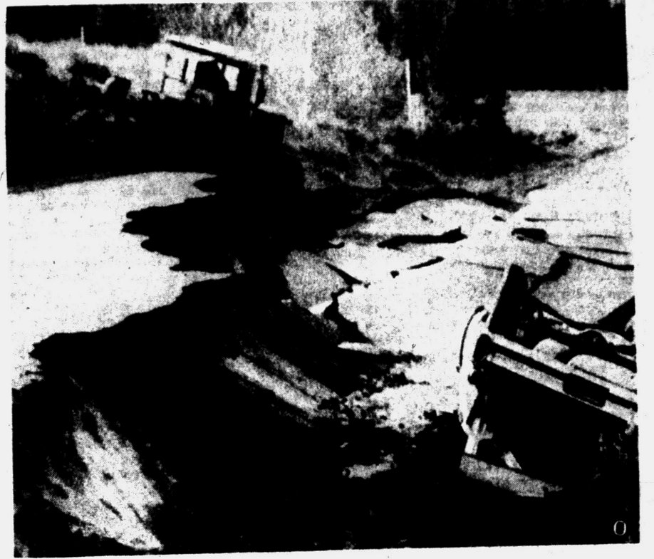
TOO EFFICIENT — An unwanted destruction job that would have taken a road crew long hours of toil was completed in seconds by a Yellowstone Park earthquake. U. S. highway 287
