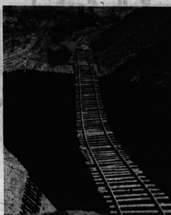
AP Photos OOPS — You might say the bottom dropped out of this railroad venture: An Iron River railroad track hangs over a cavity left when the used up Waucesa Mine caved in, isolating two men 11 days. About 10,000 tons of ore fell into the hole, which is 100 feet across and 40 feet deep.
