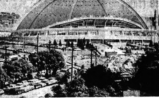
ARENA DEDICATED — Pittsburgh's new $22 million civic arena, featuring a movable dome roof, was dedicated Monday. The dome, shown partially retracted, is the largest in the world. The arena is part of a long-range development program.
