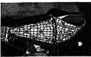
INSIDE GROUND STATION "ADONIS" AT ANDOVER, MAINE. Giant antenna inside men near rim of horn concentrates signals to Telstar in a narrow, powerful beam. In the same antenna a receiver amplifies signals coming from Telstar ten billion times.
