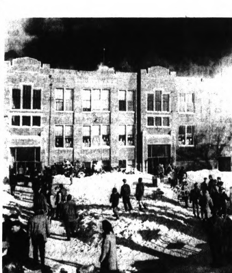
SCHOOL BURNS DOWN — This elementary school was destroyed by fire yesterday in Hayfield, Minn. Teachers and parents managed to save most of the school's equipment, but firemen were unable to save the building.
