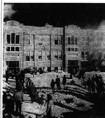
SCHOOL BURNS DOWN — This elementary school was destroyed by fire yesterday in Hayfield, Minn. Teachers and parents managed to save most of the school's equipment, but firemen were unable to save the building.
