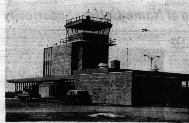
THE NEW TERMINAL — An airplane hovering over the runway completes this portrait of the new terminal building at Pontiac Municipal Airport. The $344,000 building, finished this month, is topped by a three-story tower which will be operated by the Federal Aviation Agency. This view shows the entrance to
