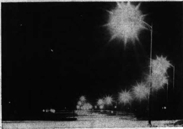
Newly installed Mercury Vapor street lights on Perimeter Road.
