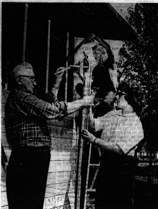
CABINS FOR CAMP MEETING — Rita Kent of 77 Westwood assists J. C. Hodge (left) as he works on cabins in preparation for the coming camp meeting at Evangelistic Tabernacle, 2800 Watkins Lake Road Thursday through July 28. High up on a stepladder Roy Linton of 1272 Schoman tightens screws at Windows.
