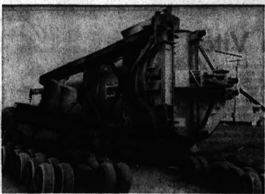
REACTOR GONE ASTRAY — The 210-ton nuclear reactor core destined for a nuclear power plant under construction by the Wisconsin-Michigan Power Co. near Kewaunee, Wis., went astray Saturday when it slipped off its transport dolly and toppled
