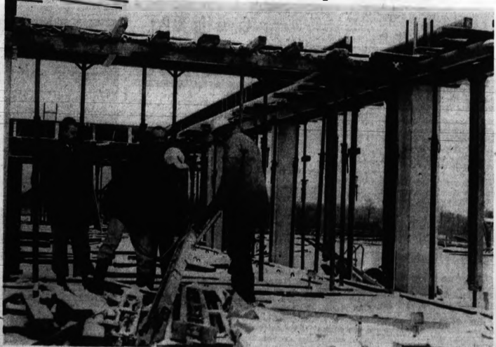
WINTER AT MSU — Despite cold and snow, building of the 11.5-million Kresge Library on the Michigan State University Oakland campus goes forward. Watching the work in near-zero weather Friday are George Karas (left), director of MSU's physical plant; and David Wilder, MSU librarian. Robert Kaminski, an engineer, and Red Krumer (right) of the A. Fredman Co. show how a new construction technique—the installation of subunits in prestressed concrete sections—will enable completion of the three decks before the outside shell is finished. Completion date of the library is Sept. 1.
