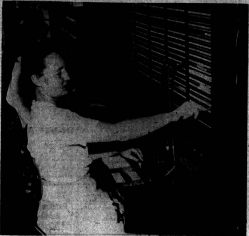
TELEPHONE SET-UP AT SCOUT CAMP —This vast switchboard is required to take care of the phone calls to and from the 5,000 Girl Scouts at National Girl Scout Roundup at Highland Recreation area. Here Pontiac operator
