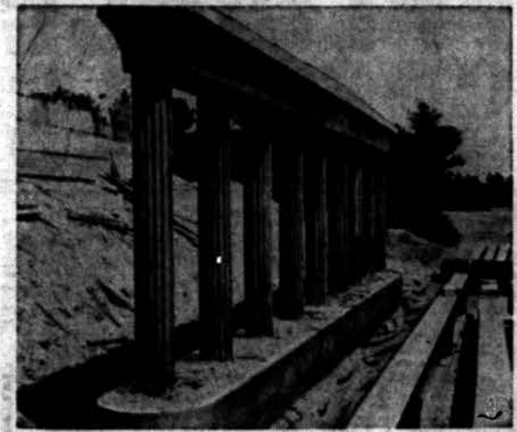
PAST PRESENT — No remnant of a past civilization, these fluted columns now support a bridge on newly located Route 134, which crosses the Mid-Cape Expressway at Dennis, Mass.
