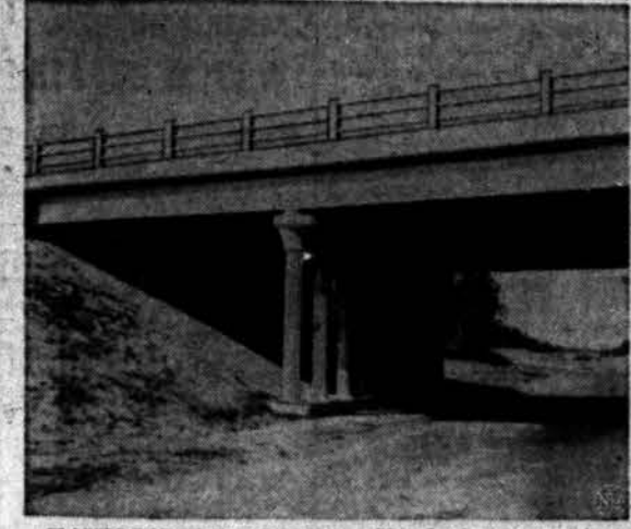
CLASSIC TOUCH FOR BRIDGE — Fluted columns, reminiscent of Roman ruins, support this new bridge across the Mid-Cape Expressway at Dennis, Mass. Relocated Route 134 is carried by the structure.
