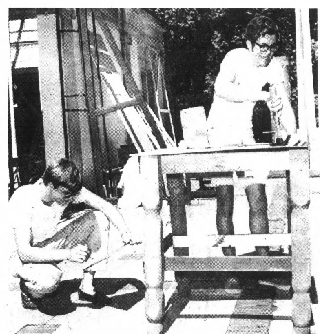
Helping to turn the cement stage of the Cranbrook Greek Theatre into a fairyland setting are, from left, Jim Locker of Birmingham, and Harold Green of Farmington. Their project at this moment was the construction of a throne for King Philip of Cardocia.
