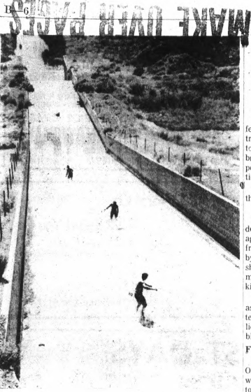
DEADLY FUN—It looks like fun, but it could be deadly, warns the U.S. Bureau of Reclamation. The Rocky Coulee Chute near Moses Lake, Wash., ends in rough concrete breakers to slow the water. It takes only 15 seconds to travel the 935 feet from the top to the bottom. Hitting the breakers could end in injury or death, the bureau says. One drowning occurred this summer as boys slid the Esquatzel Chute near Pasco, Wash.
