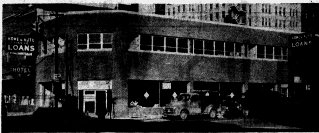
FIRM TRANSFERS OFFICES —New headquarters for the Home & Auto Loan Co. is this modern, brick and steel structure at 7 N. Perry St. into which the company's staff of 11 moved yesterday. The air-conditioned building features five private consultation rooms in addition to other expanded facilities for customers. Established
