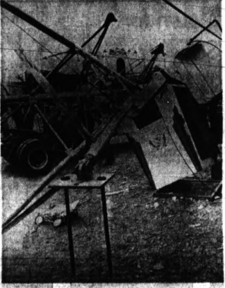
TOPPLED TOWERS — Huge stakes that braced a cable car "Sky Lift" ride at the Nebraska State Fair in Lincoln were uprooted yesterday, dropping passengers in gondolas more than 30 feet into the crowd below. Two persons were killed and 48 injured in the mishap. One of the toppled towers is shown where it crushed the ticket booth for the ride.
