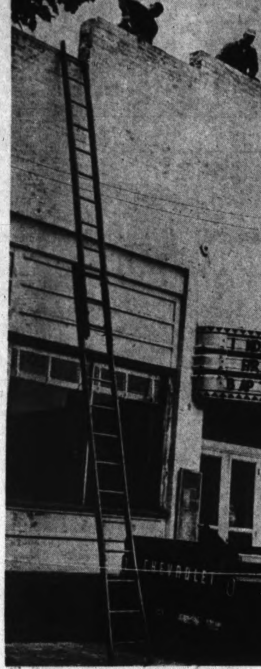
GETS NEW LOOK — Workers are shown removing loose concrete from the State Theater at 101 S. Broadway St., Lake Orion, which will be the new headquarters for the Lake Orion Youth Center after renovation of the building is completed.
