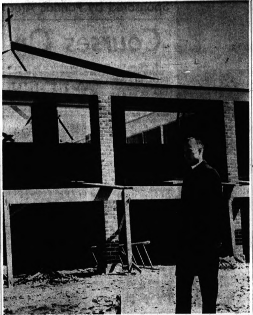
GOING UP —Pastor Robert Franklin of 2364 Mulberry, Bloomfield Township, looks over the construction of the new Incarnate Lutheran Church going up on Opdyke just north of Square Lake. The congregation is presently worshipping in the Eastover Elementary School, Bloomfield Township.
