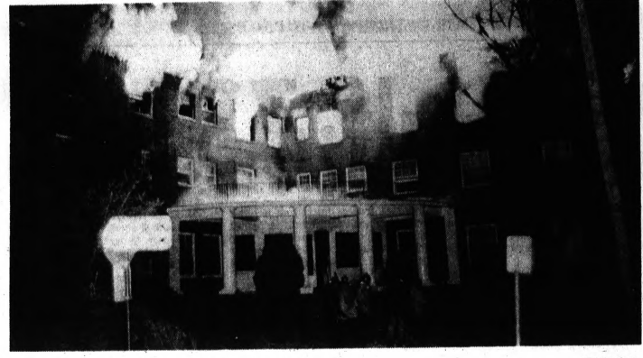
BLAZE KILLS 12 — Fire swept through a Kansas City, Mo., apartment building early today, killing 12 persons. A number of residents were carried down ladders from the second and third floors, and some escaped down three of the four fire escapes on the building.
