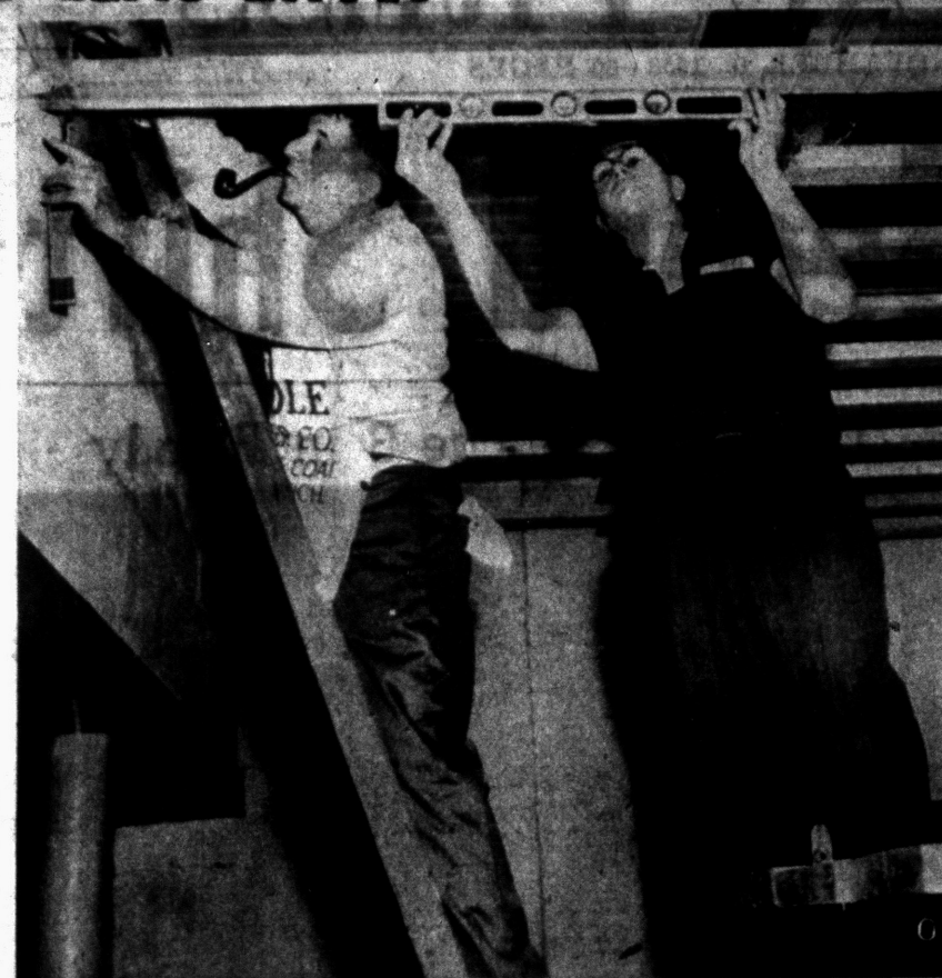
FINISHING TOUCHES—Members of the West Pontiac Kiwanis Club are shown here putting the finishing touches on a winterizing project at the Boy Scouts' Camp Agawam, near Lake Orion. The club has spent about a month insulating the camp's main hall. The value of the building was raised an estimated $3,000 by the Kiwanis project. Pictured here, Jim Scribner, one of the club's directors, (left) and Bill Brandt, president elect, work on insulating the ceiling. The project was completed this weekend.
