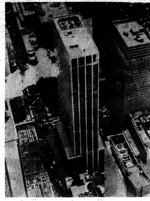
VIEW FROM THE SKY—This is the new 45-story J.C. Penney building in New York. Penney's new central office provides a more efficient base from which to speed merchandise to nearly 1,700 stores and their millions of customers.
