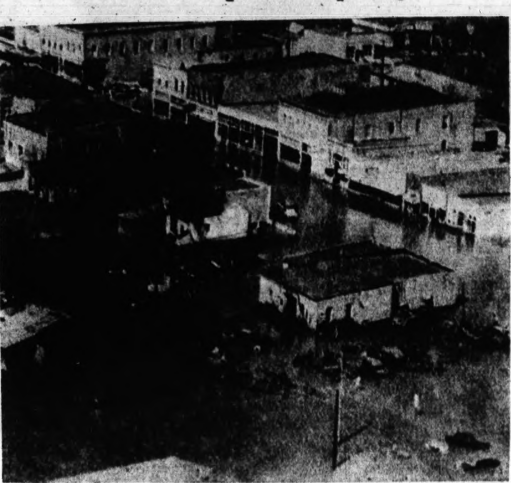
VERNON DOWNTOWN — Floodwaters of Black Vermilion Creek cover part of the Frankfort, Kan., business district a foot deep Monday as a result of a runoff caused by the spring thaw melting leftover snow. About 40 blocks were affected by the overflow.
