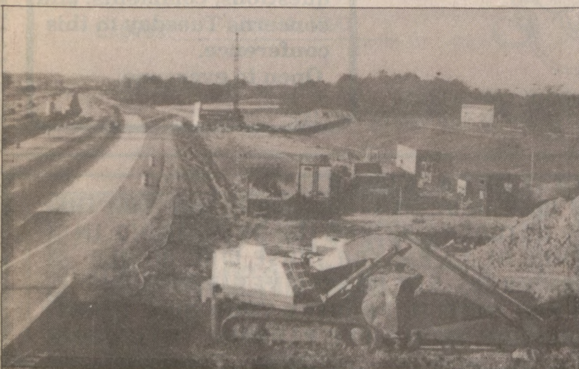
Construction on I-75 before the University Drive exit is expected to be completed by October 31, 1991.
