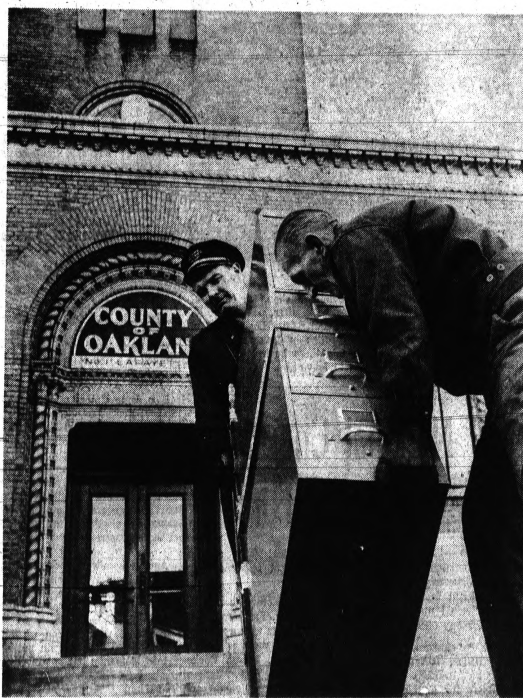
MOVING OUT — County offices at 1 Lafayette St., downtown, are in the process of being moved to the new courthouse wing at the County Service Center on Telegraph Road. The downtown building will be closed Tuesday and business will resume at the wing the next day. This will complete the county's move of facilities from downtown Pontiac. Movers are John Lytle (left), and Larry Washburn of Allied Van Lines, Inc.
