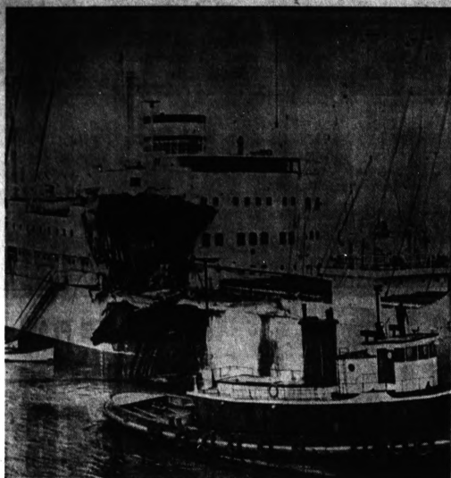
CRUSHED AMIDSHIPS —The Norwegian freighter Berganger is severely damaged in its center section following yesterday's collision in San Francisco Bay with the Liberian tanker Intercontinent. The freighter was hit
