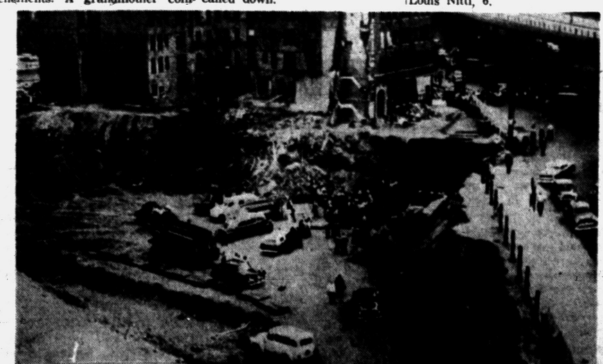
SIX CHILDREN LOST THEIR LIVES — Rescue workers probe area of cave-in which snuffed out lives of six children late yesterday afternoon near the Brooklyn end of the Williamsburg Bridge
